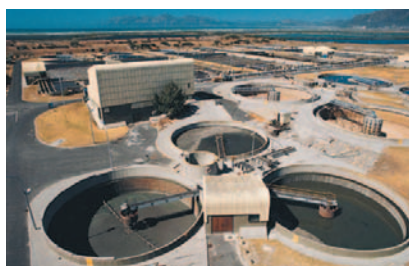
Example of remote communications application
